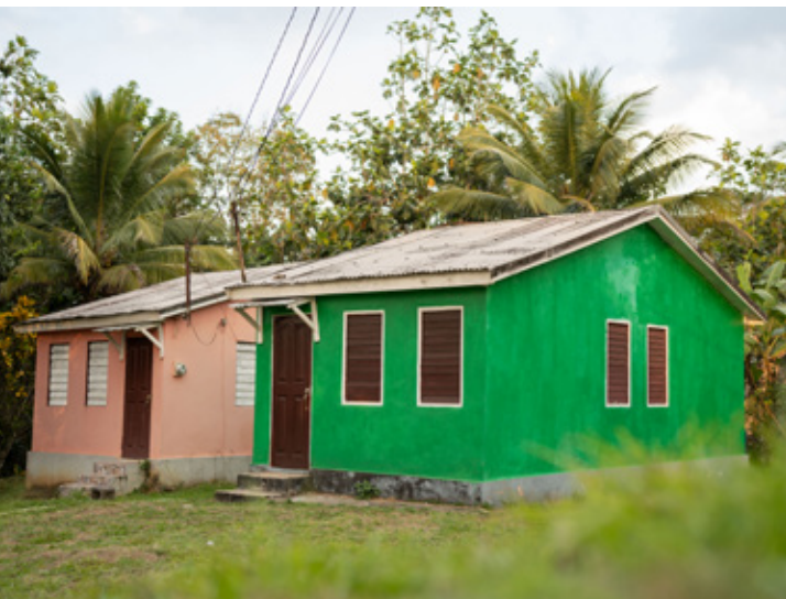
One of the first units to be built in Bethel Town Housing Scheme
